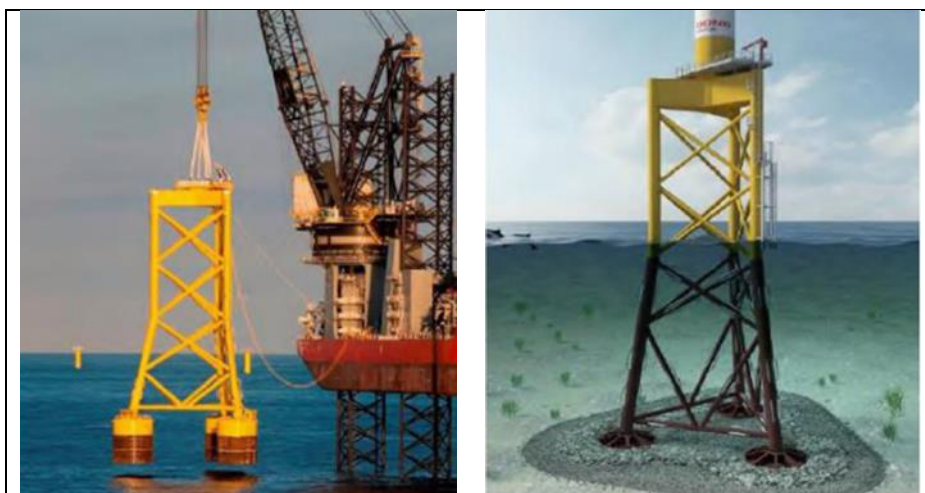
Figure 3.6. Suction bucket jacket (SBJ) foundation [Source: Ramboll]
