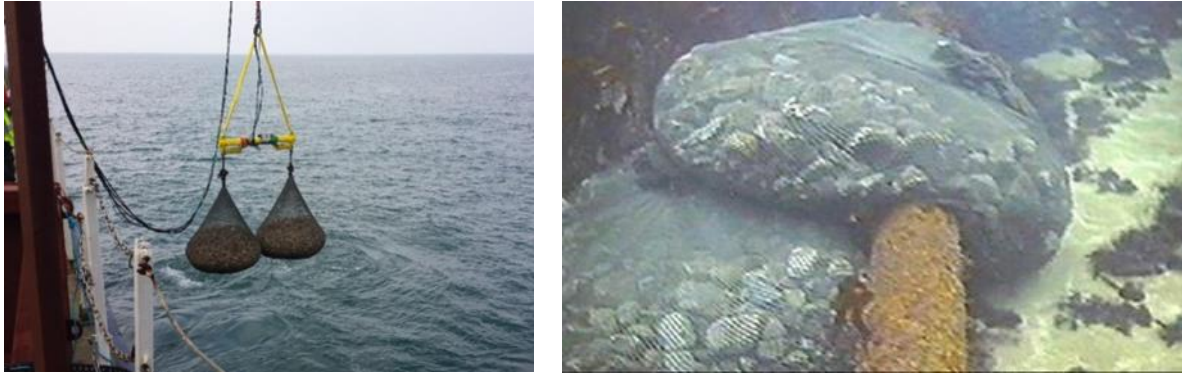
Figure 3.21. Method of constructing and laying rock bags on a cable line [Source: bluemont.com.au]
