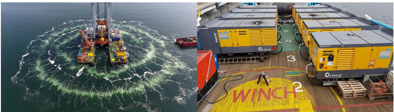
Figure 7.35: Illustration of a DBBC mitigation system (Left: in effect; Right: compressors for creating the air pressure) (Source: hydrotechnik-luebeck.de ).
